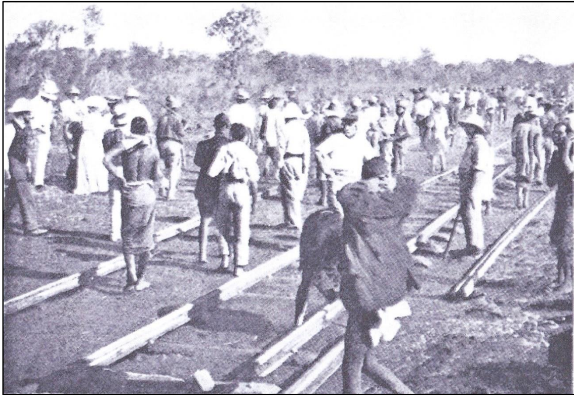
Unballasted track being laid at the rate of a mile a day north of Machudi
